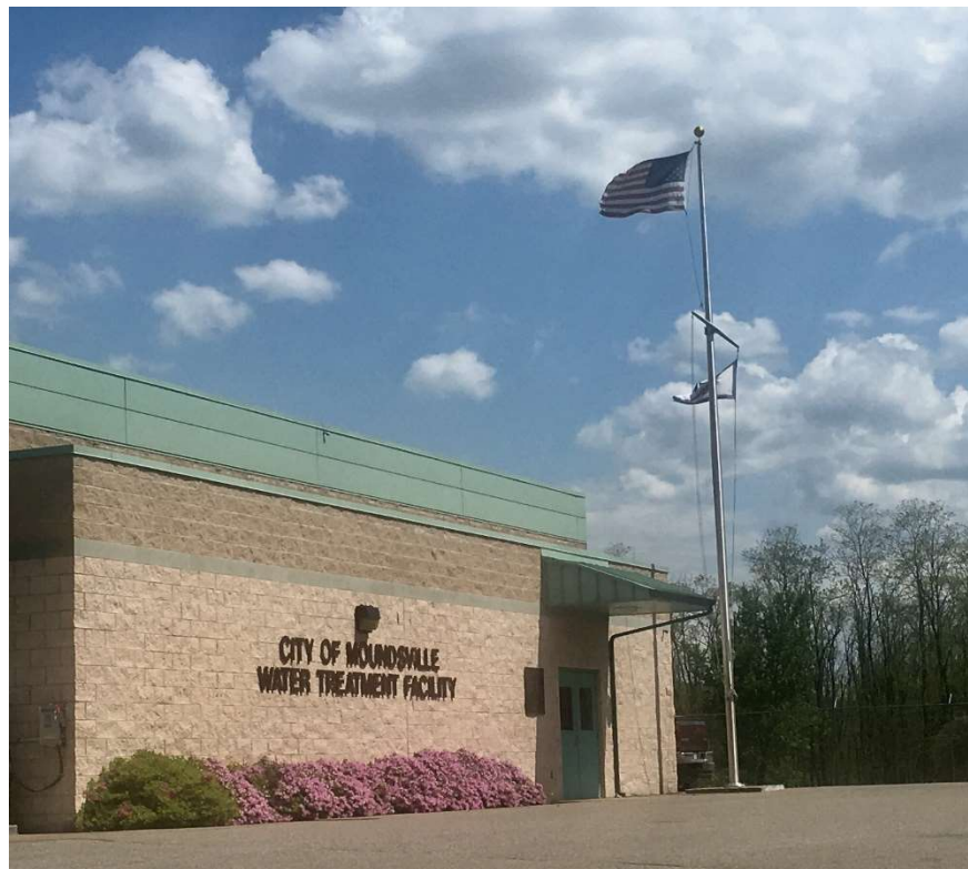
Water Treatment Plant - Front View along Ohio River
